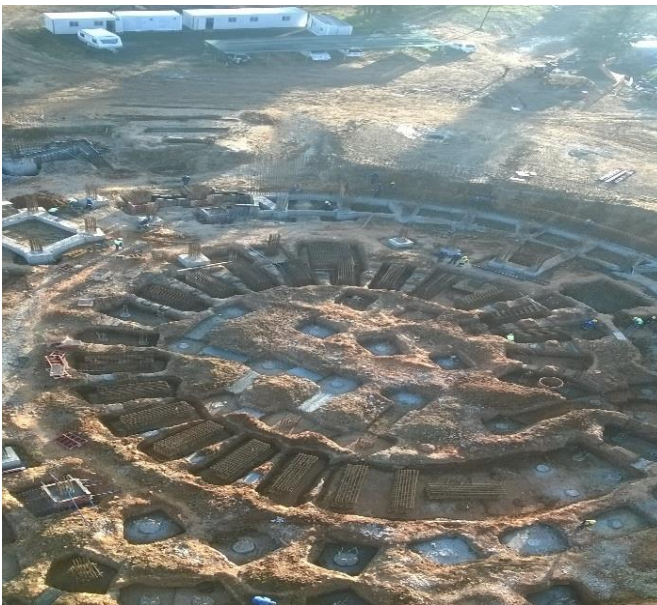
Piling and Ground Beams
